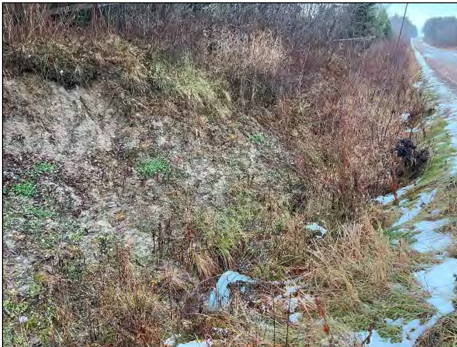
PHOTO 2 – SW2 – Upstream side of Culvert (Fall 2023, Facing East)
