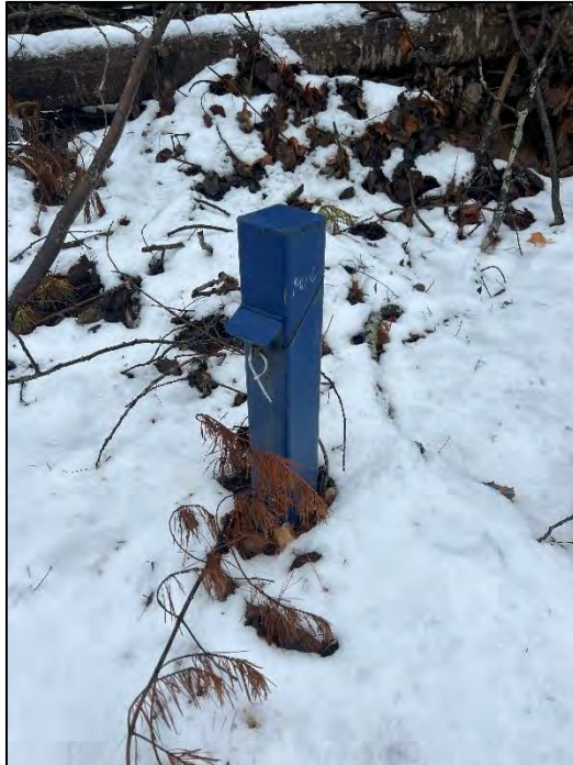
PHOTO 9 – MW6 – (Fall 2023, Facing South)
